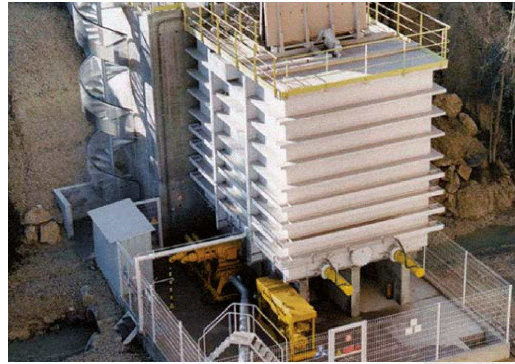
Co-incineration of alternative fuels in the cement plant of Lafarge in Le Teil, France
